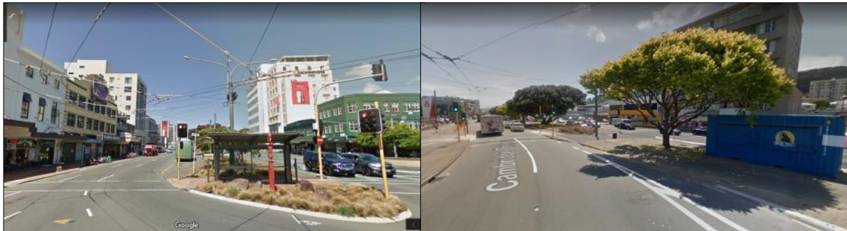
Figure 32. Kent and Cambridge Terraces view from Courtenay Place (left). View from Basin Reserve (right)
