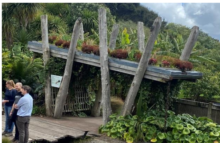
Figure 9. A green roof at the Auckland Botanic Gardens, forming part of the Auckland Sustainable Stormwater Trail. Photo: R. Simcock (with permission).
