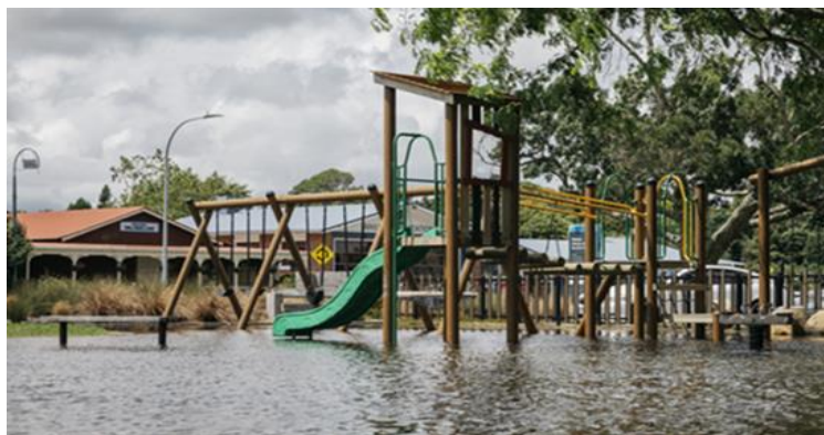
Figure 3. An urban park acting as a stormwater detention area in Auckland following the February 2023 flooding events described in Section 1. Photo: Auckland Council (with permission).
